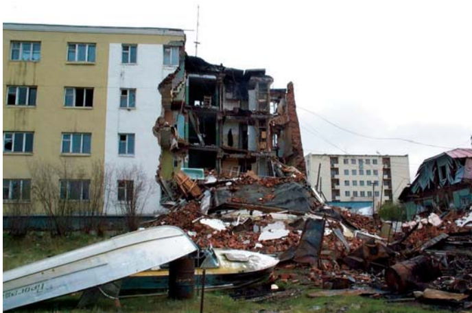
Figure 4. Section of the residential building in town Cherskiy, lower Kolyma River valley, collapsed in June 2001 as a result of weakening of the foundation built upon permafrost. Although there is still a debate whether the climatic change or improper management of the construction caused warming and thawing of the frozen ground underneath the building, the accident illustrates the potentially detrimental impact of permafrost degradation, whichever is the factor that caused it. Photo: by V.E. Romanovskiy.
